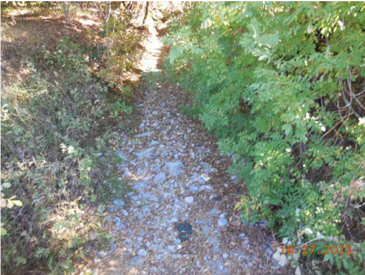
Figure 1. Image looking upstream of Pruitt Creek at Old Redwood Highway on October 27, 2023.
