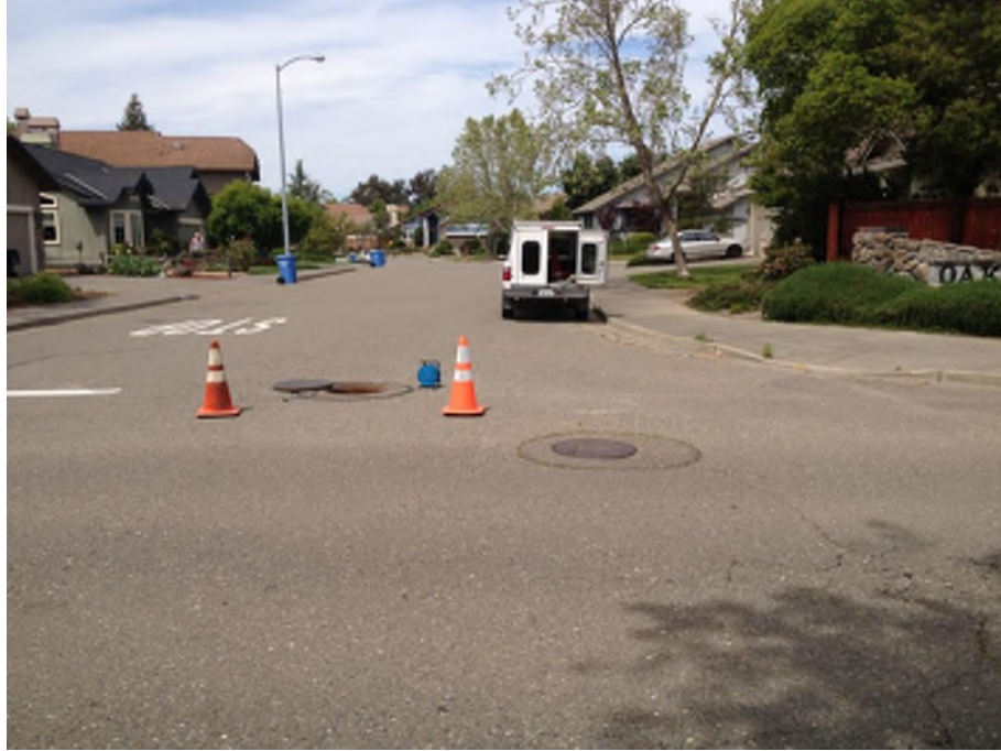
S130B on Gridley Dr Windsor, Ca, Looking North
