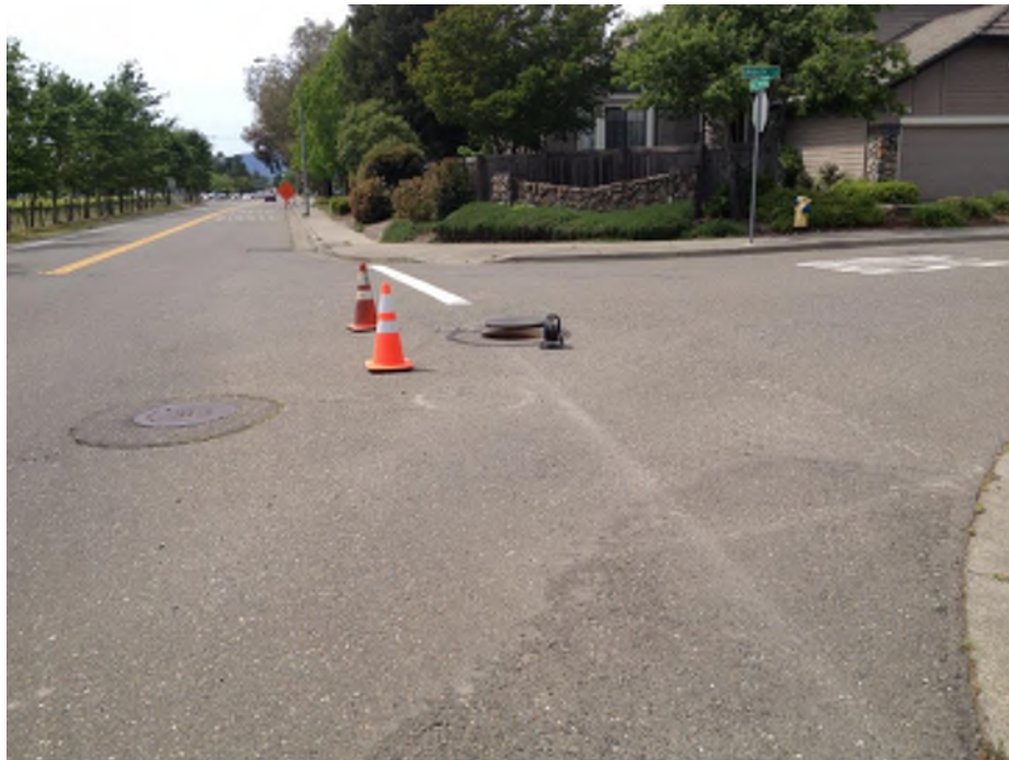
S130B on Gridley Dr, Looking west on Shiloh Rd, Windsor, Ca
