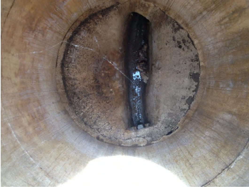
6.5 ft from rim to bottom, 8-inch sewer lateral
