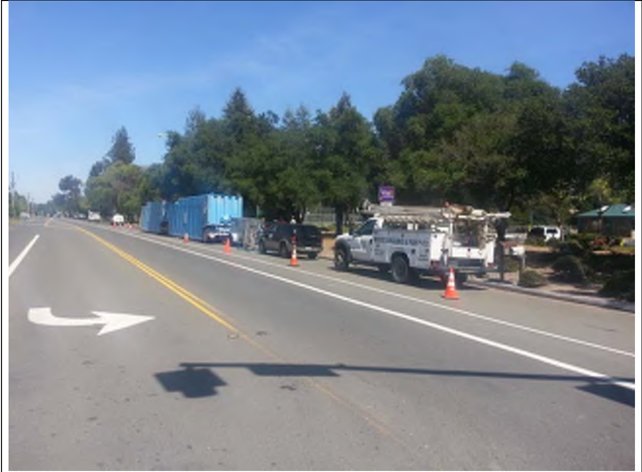
Baker tanks staged along Old Redwood Hwy.
