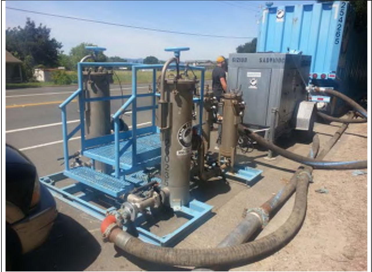
Bag filters used for sediment removal prior to discharge of water to sanitary sewer.
