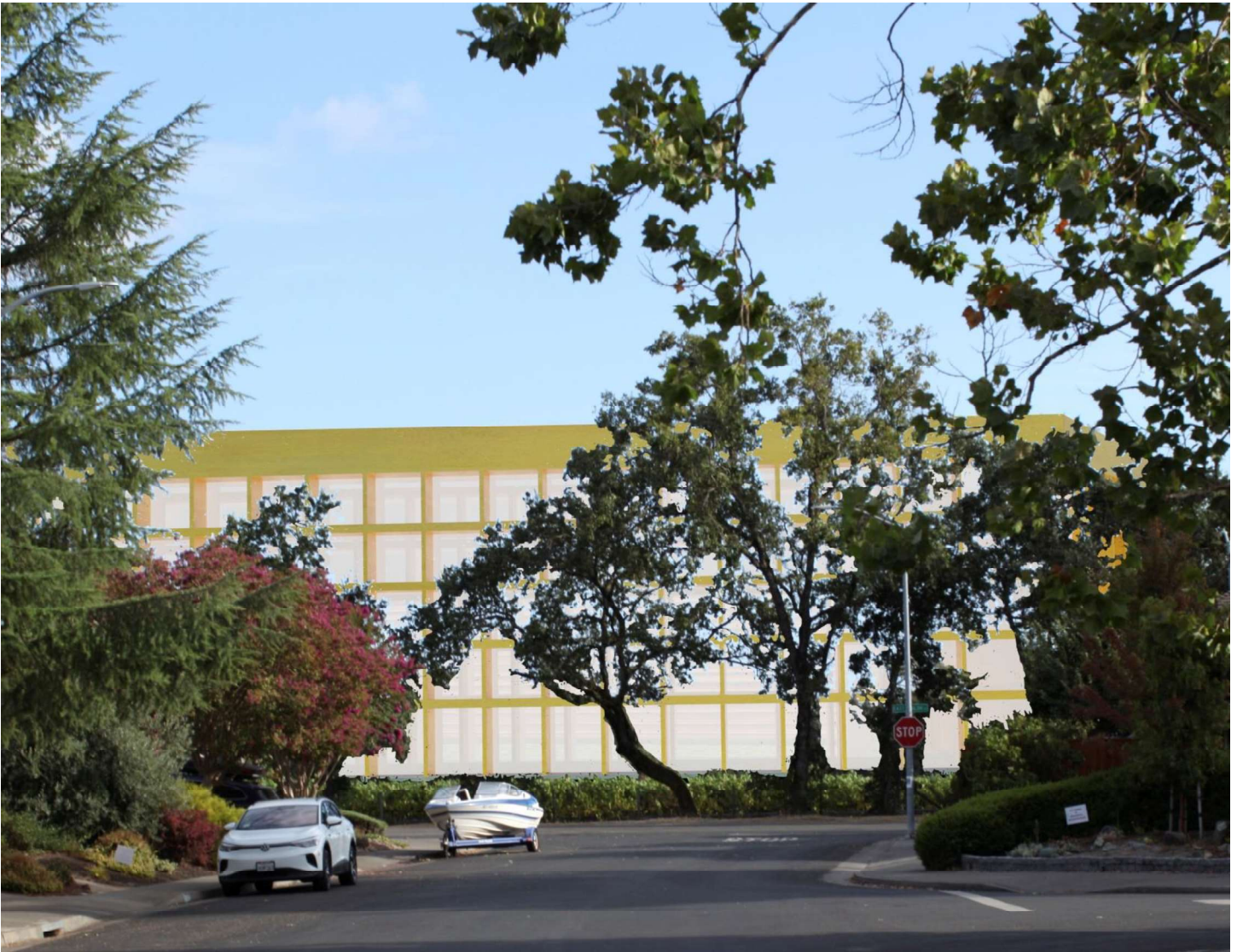
[ Shiloh Resort Hotel viewed from the Oak Park neighborhood: “less than significant visual impact.” ]
