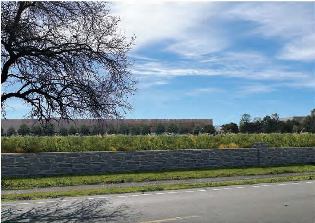
View of Alternative A from Shiloh Road with Reservoir
