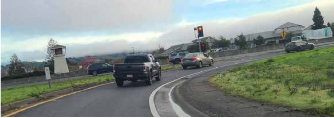
Highway 101 Southbound On-Ramp
