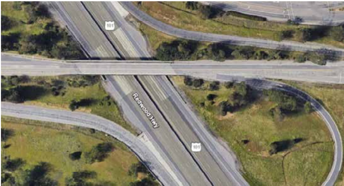
Road Damage on Shiloh Overpass and Ramps
