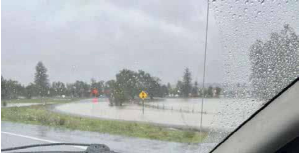
Highway 101 Northbound Off-Ramp Flooded (Closed) in November 2024
