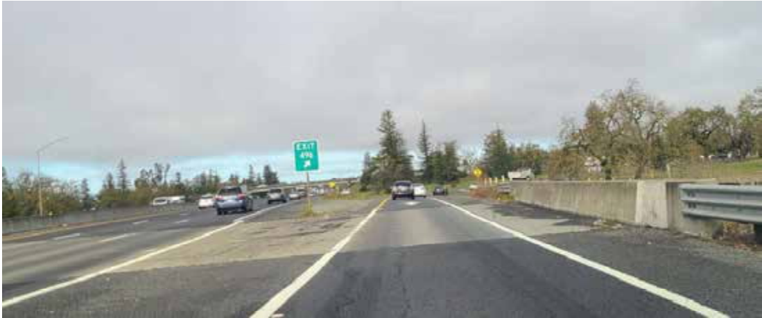
Highway 101 Northbound Off-Ramp
